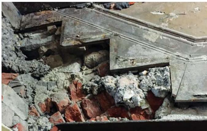
Degradation of masonry and plaster due to moisture
